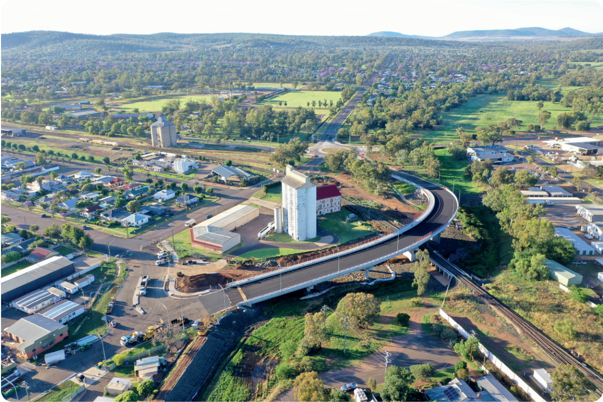
Image credit: Daracon. Gunnedah Bridge Infrastructure Project.
