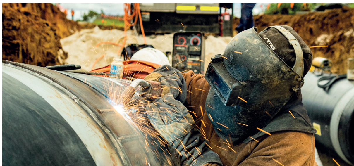
Image credit: Vaughan Civil Pty Ltd – Prospect South to Macarthur (ProMac) Package 17.
