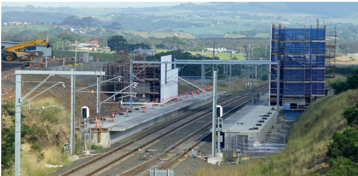
Image credit: Haslin Constructions Pty Ltd - Shellharbour Junction Railway.
